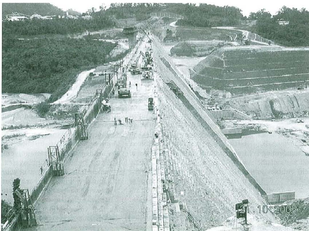
Sg. Kinta Dam under construction. View towards the left abutment.
