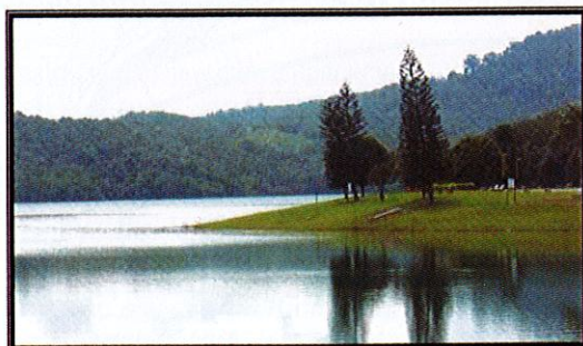
View of Existing Mengkuang Dam Storage Reservoir
