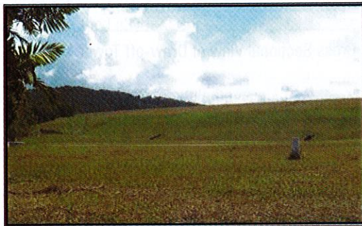
View of Existing Dam Embankment
