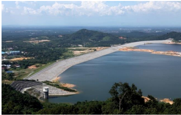
Figure 3 - Panoramic View of the Mengkuang Dam
